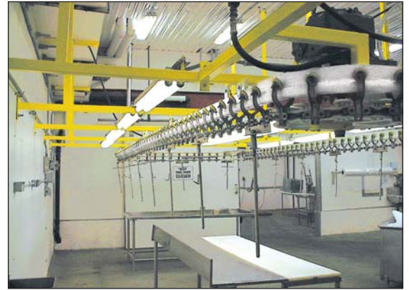
Poultry Processing Facility
